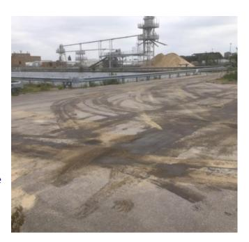
Due to the nature of the damages we immediately arranged for a Senior Civil Engineer, who specialises in resurfacing, to attend site and inspect the damages. He was able to confirm the contaminated filter bed had now been rectified and was fully operational; however the resurfacing works had yet to commence. They measured the affected area at a total of 578m2 and that this would require planning to a depth of 40mm.
