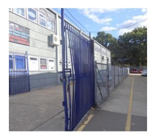
site. Upon inspection the surveyor confirmed the gate frame had been bent and that the vertical metal railings were out of alignment, the damage was consistent with an impact and was to the right-hand gate only.
