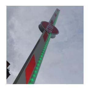
At the point of our instruction repairs had already been completed and we instructed one of our Surveyors to attend. From the images provided the Surveyor noted that the boom arm, which had already been installed, was a different design to the one in place at the time of the incident. The arm now had LED lighting to the underside, which appeared to be an upgrade. In addition, the signage had been replaced.
